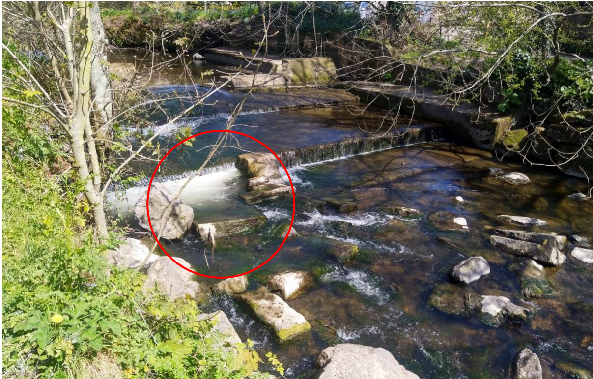
Figure 19 Looking upstream to the weir in Figures 17 & 18. A notional jumping pool has been created to ease the first step (red circle), but overall insufficient to allow good upstream fish passage. SY 12969 88498
