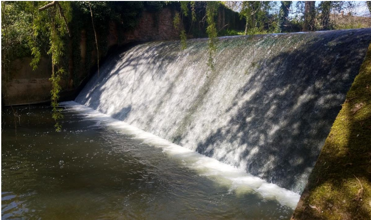
Figure 24 School Weir seen from downstream. At around 3m high, it is beyond the scope of any salmonids to ascend without help. SY 12790 87895
