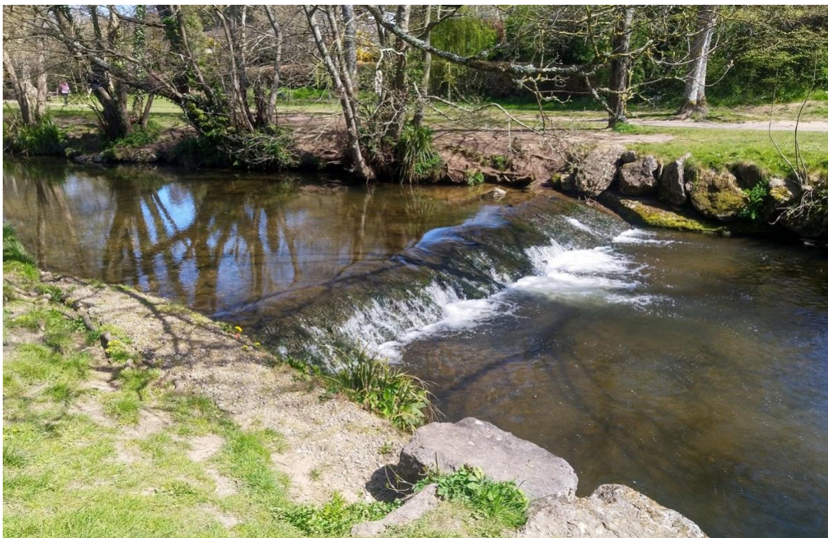
Figure 20 A slightly more conventional Check Weir. Though not impassable, it still presents an unnecessary stress and delay to upstream and downstream migration. The impounded reach above is also severely lacking habitat diversity caused by the impoundment. Removal or significant alteration is recommended. Adding large woody material (LWM) would also be beneficial. SY 12880 88343
