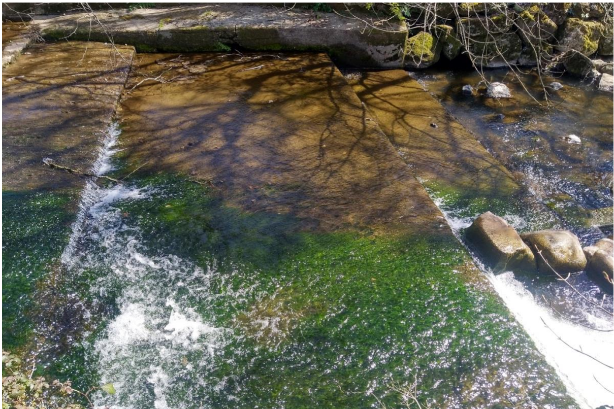
Figure 18 The three shallow steps downstream of the weir in Figure 17. In low to medium flows, there isn't enough water for fish to swim upstream. SY 12969 88498
