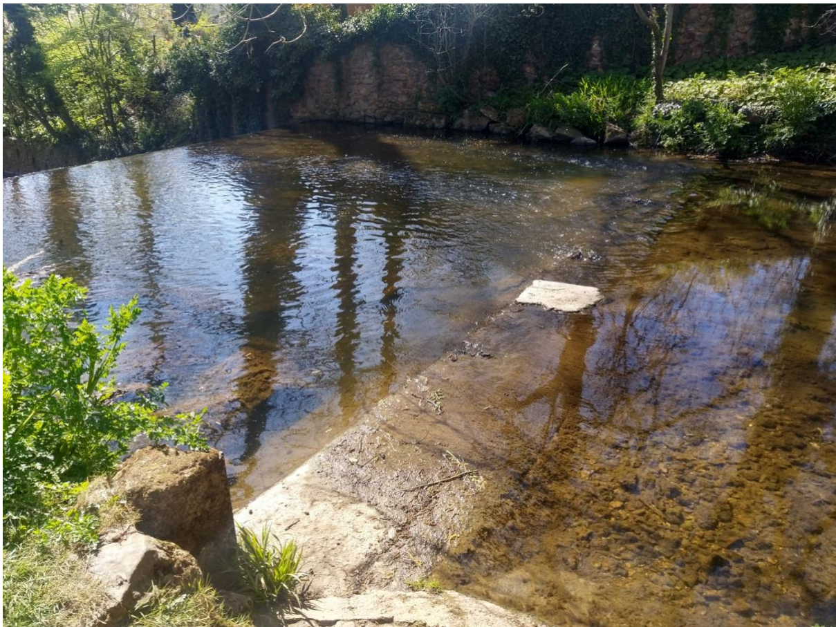
Figure 26 The old mill weir, approximately 10 metres up from School Weir. With lowering and notching, this could form the first part of a cascade to ease passage while limiting the lowering of the river upstream. SY 12790 87895
