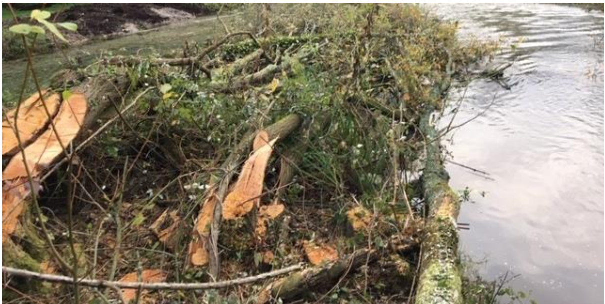
Figure 33 Hinged willow on the River Test. Hazel, small willows and small alders can be hinged into a river, creating diversity of flow and in-stream cover for fish. The trees are hinged in a similar manor to hedge laying, where the tree is partially cut through at the base and laid into the margins. Chestnut stakes and fencing wire can be used to secure the trees in place. Willow will survive perfectly well even with 70% of the branches submerged; however, hazel and alder should be laid to retain much of the structure above water level.
