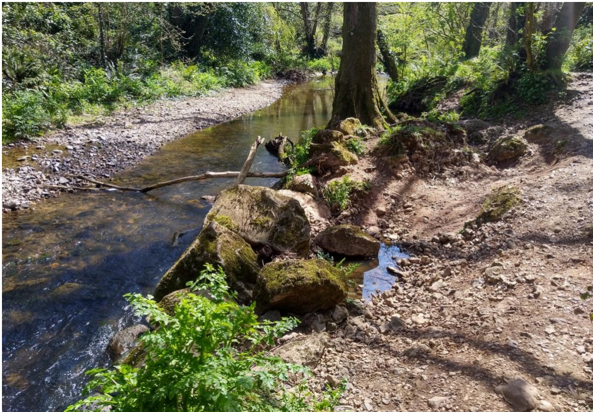
Figure 8 Erosion is beginning to cut around the back of this tree. Considering the straightness of the channel downstream, this could be a place to encourage a bend by manipulating the boulder weir immediately upstream. Felling the tree across the channel could arrest flows and help with the diversion. SY 13279 88875
