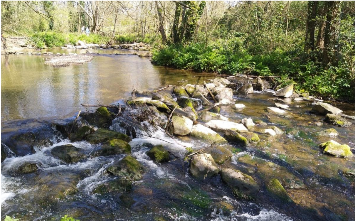
Figure 7 A cascade of several boulder weirs. SY 13279 88875
