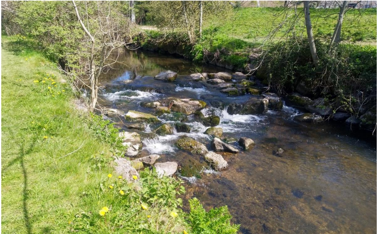
Figure 21 A better looking rubble weir, though still an unnecessary impediment to natural river function and fish migration. With room on both banks, the gradient could be reduced through meandering rather than an unnatural step. This would restore a lateral scour pool and riffle sequence, good for all salmonid life stages. SY 12863 88312
