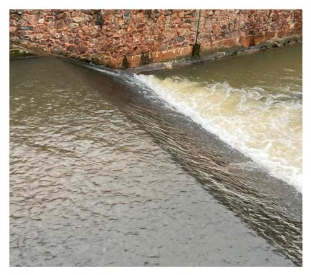
Figure 7 Sloping weir immediately downstream of the ford
