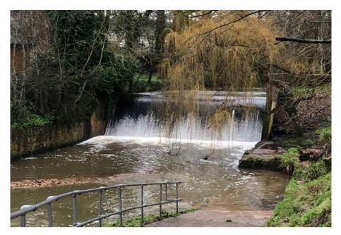
Figure 5 School weir from downstream with access ramp and bedload accumulation
