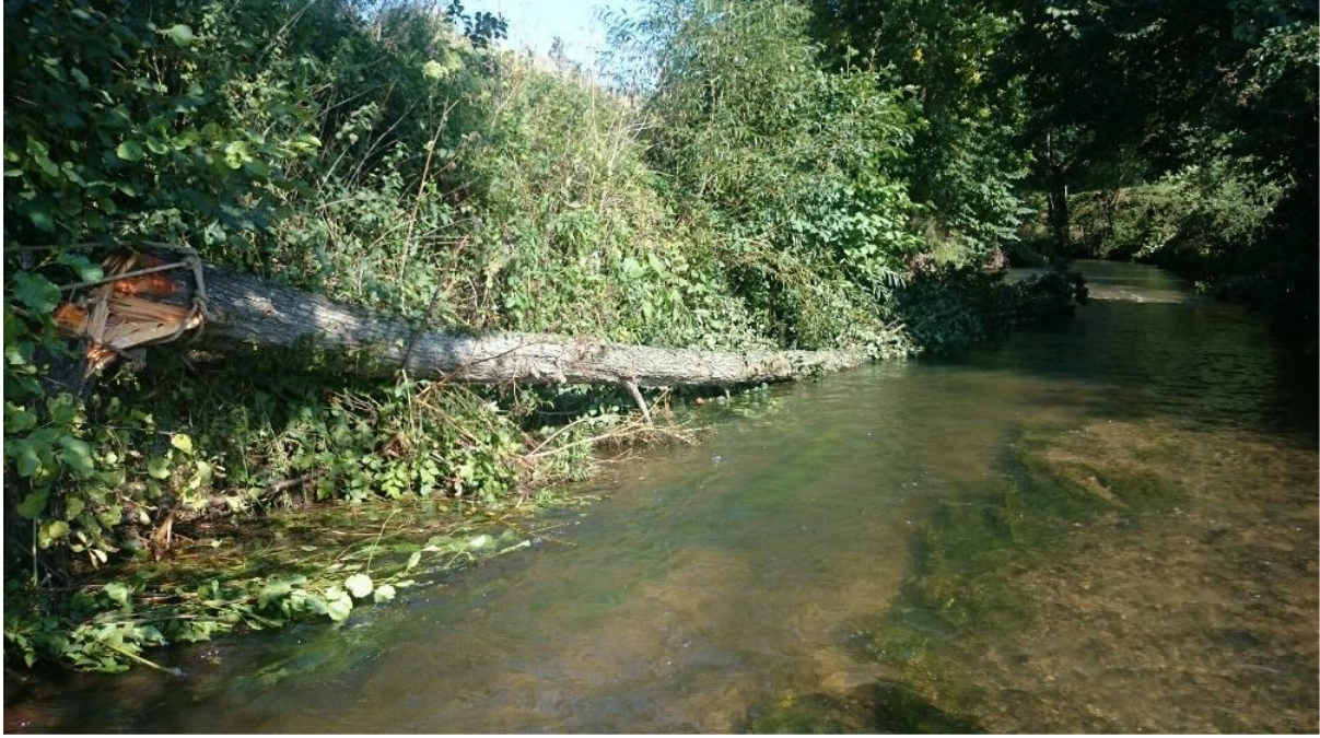
Figure 10: An example of a hinged alder tree laid into the margins of a spate river. Rope has been used to secure the tree as a redundancy, however steel wire may also be used where there is greater flood risk concerns.
